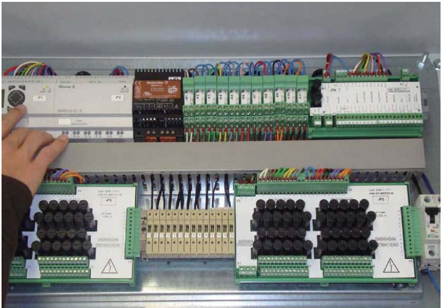
阀门可经由一个控制柜来连接不间断电源 Valves can be connected via a control cabinet, with an uninterruptible power-supply
